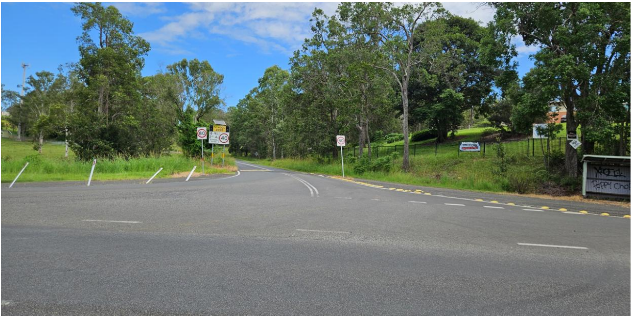
Photograph 8.9 Bentley Road/Manifold Road intersection (looking south-west)
