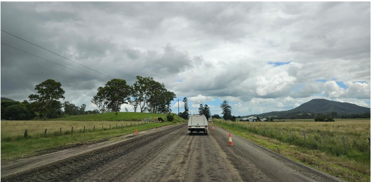
Photograph 8.2 Roadworks in Bentley Road (looking west)
