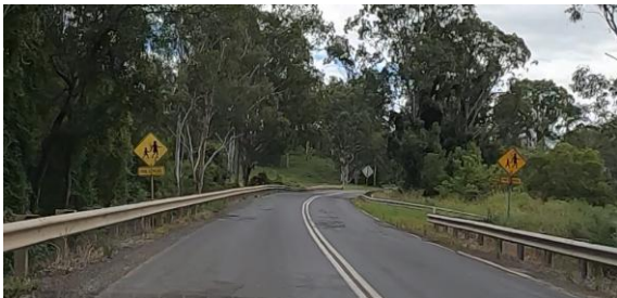
South approach (northbound traffic)
