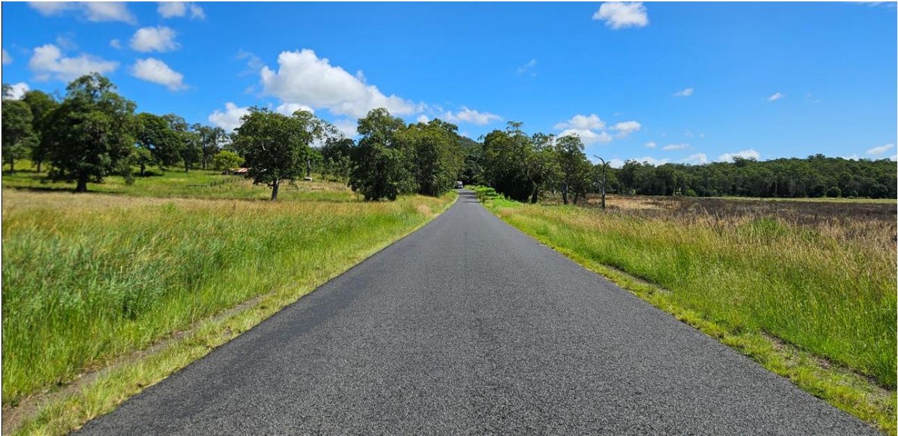
Photograph 8.11 Straight section of Naughtons Gap Road (looking south)
